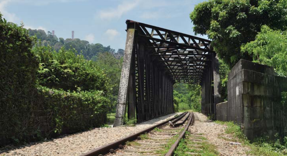
Upper Bukit Timah Truss Bridge along the 24km Rail Corridor.
